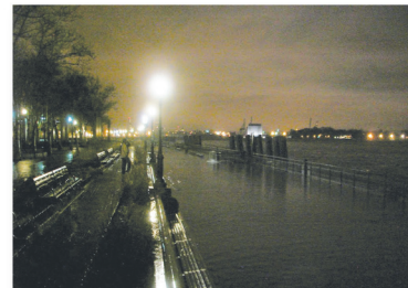
The promenade at the Battery was also completely inundated from the flooding event. The seawall is pictured here on the right.
