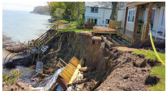
Coastal Infrastructure impacted by erosion in Monroe County. Image credit: Mary Austerman, New York Sea Grant. 2017 Coastal Flooding Survey Project
