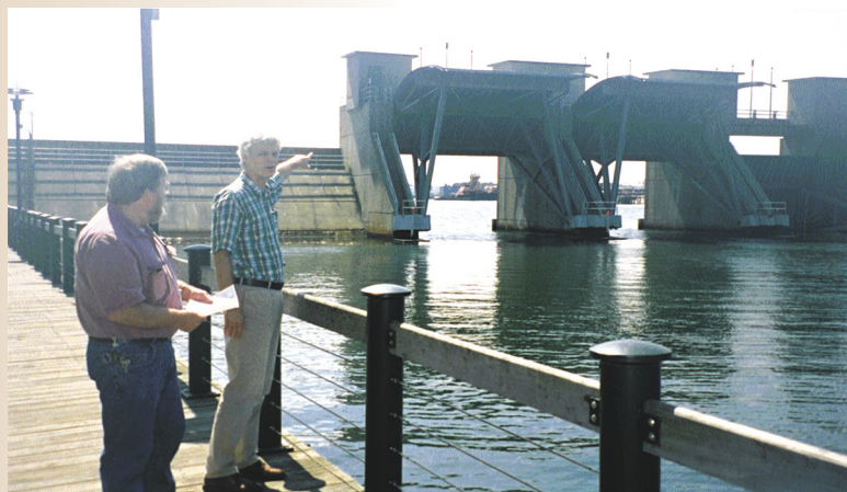
Co-investigators Roger Flood (l.) and Robert Wilson (r.) view the three Tainter gates at the Fox Point Hurricane Barrier in Providence, RI. Others working with the research group are Douglas Hill, Brian Colle, Frank Buonaiuto and several students. Photo by Douglas Hill
