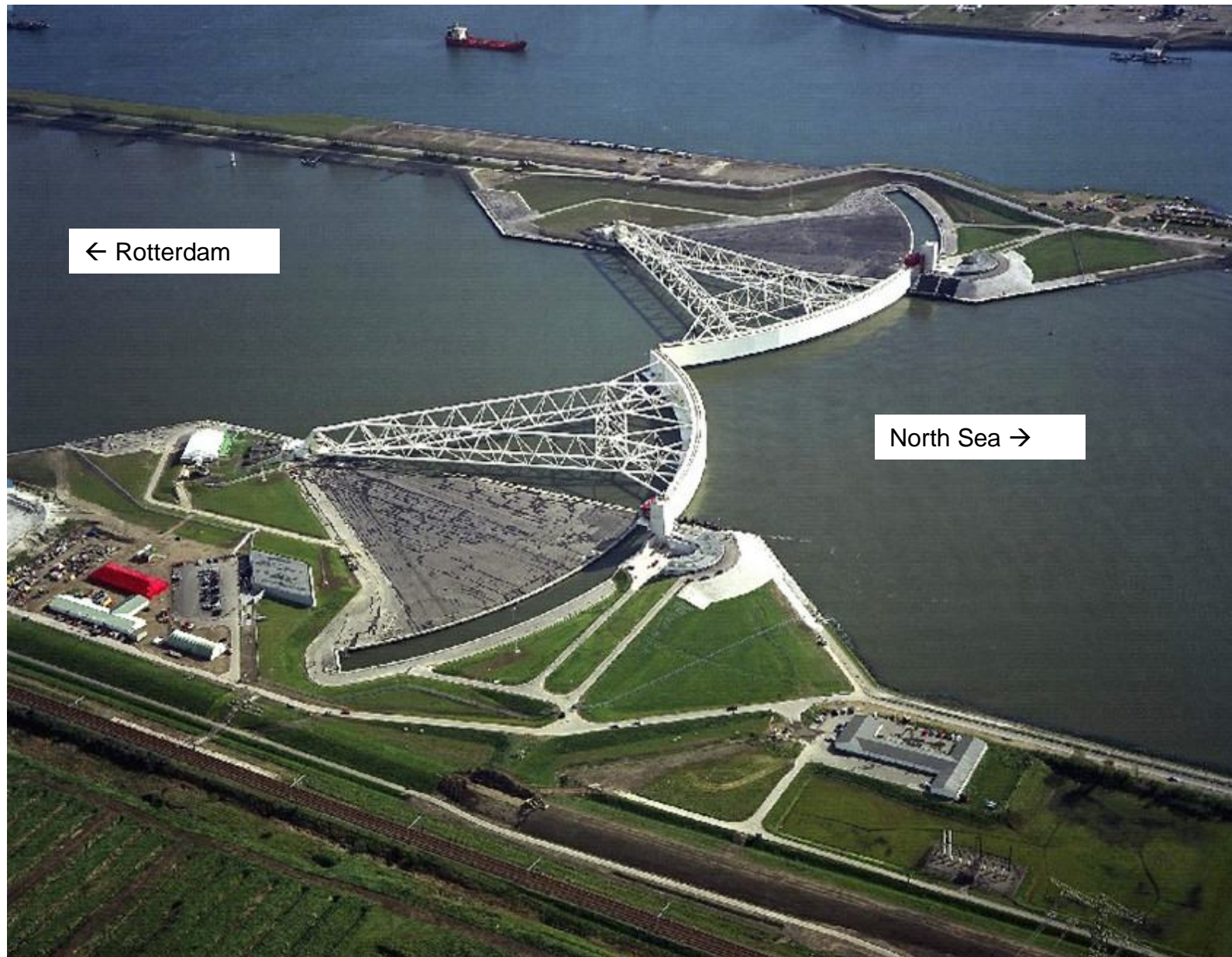
Delta Works, the Netherlands. Twin sector gate barriers (Taintor Gates) protect the port of Rotterdam, the world's largest, against North Sea storm surges. The gates are shown closed in the storm surge position. 42 Normally the gates are kept open, rotated back into their parking areas.
